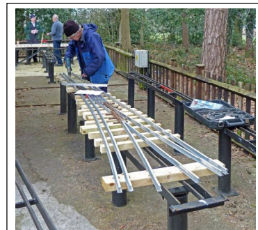
Photo Paul Archer. Derek Tulley constructing the facing point.
