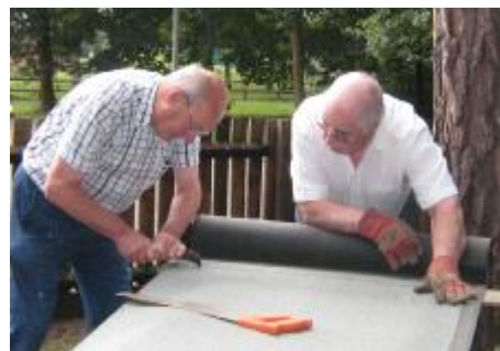
Derek having got used to the taste and feel of bitumen (see issue 14) has proceeded to re-felt the old carriage shed roof. Keith is here cutting the lengths of roofing felt while David is – well, sort of leaning on it. Photos JRK
